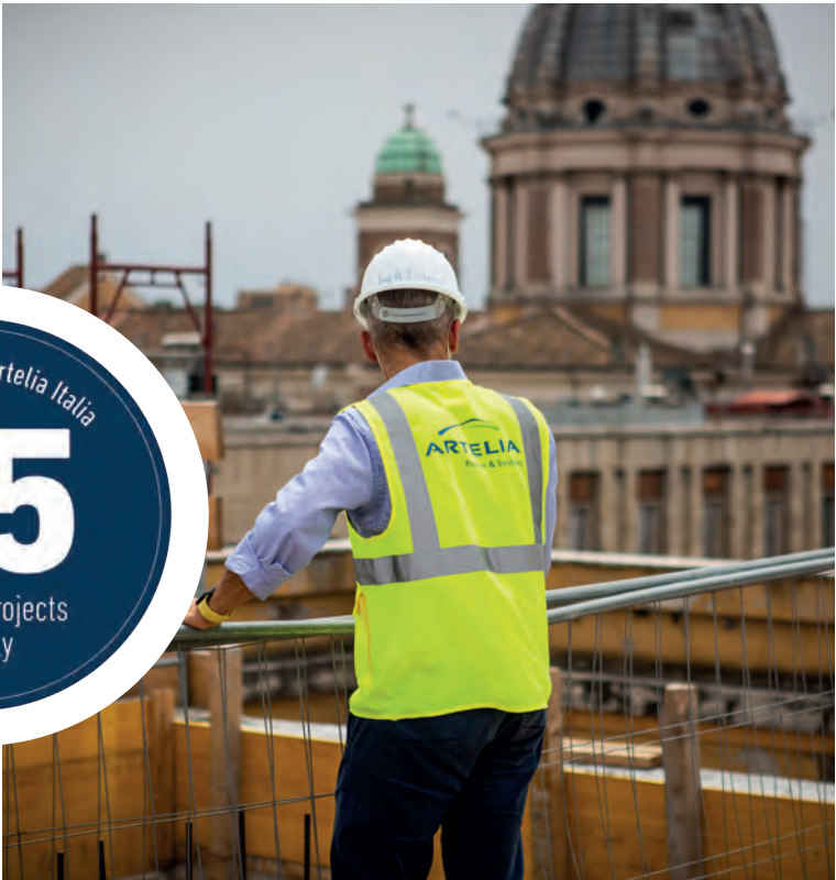
Bulgari Hotel Roma - construction site picture from the terrace - Rome, 2019
